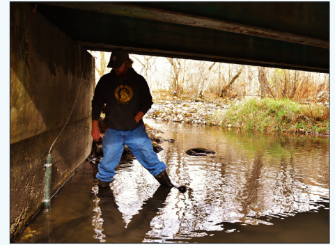
Installing a Gauging Station
