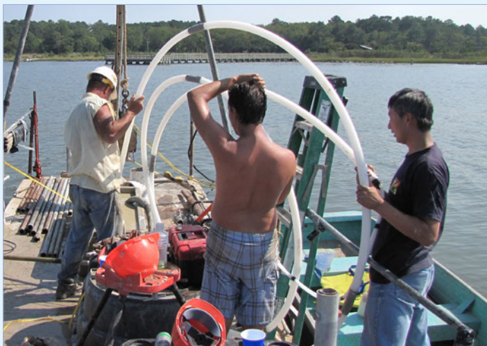
CMT Systems were Installed Below the Bay Bottom to Monitor Submarine Groundwater Discharge
