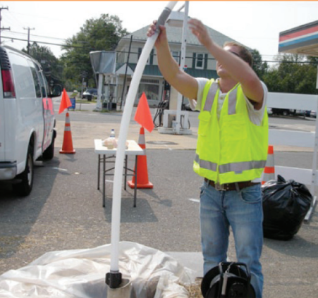
CMT System being installed in a monitoring well
