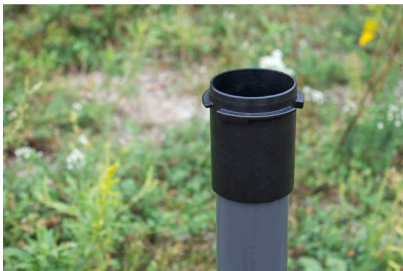
Figure 6-3 Install the Well Cap Base
