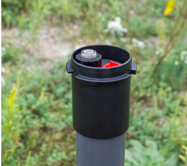
Remove Existing Levellogger Installation
