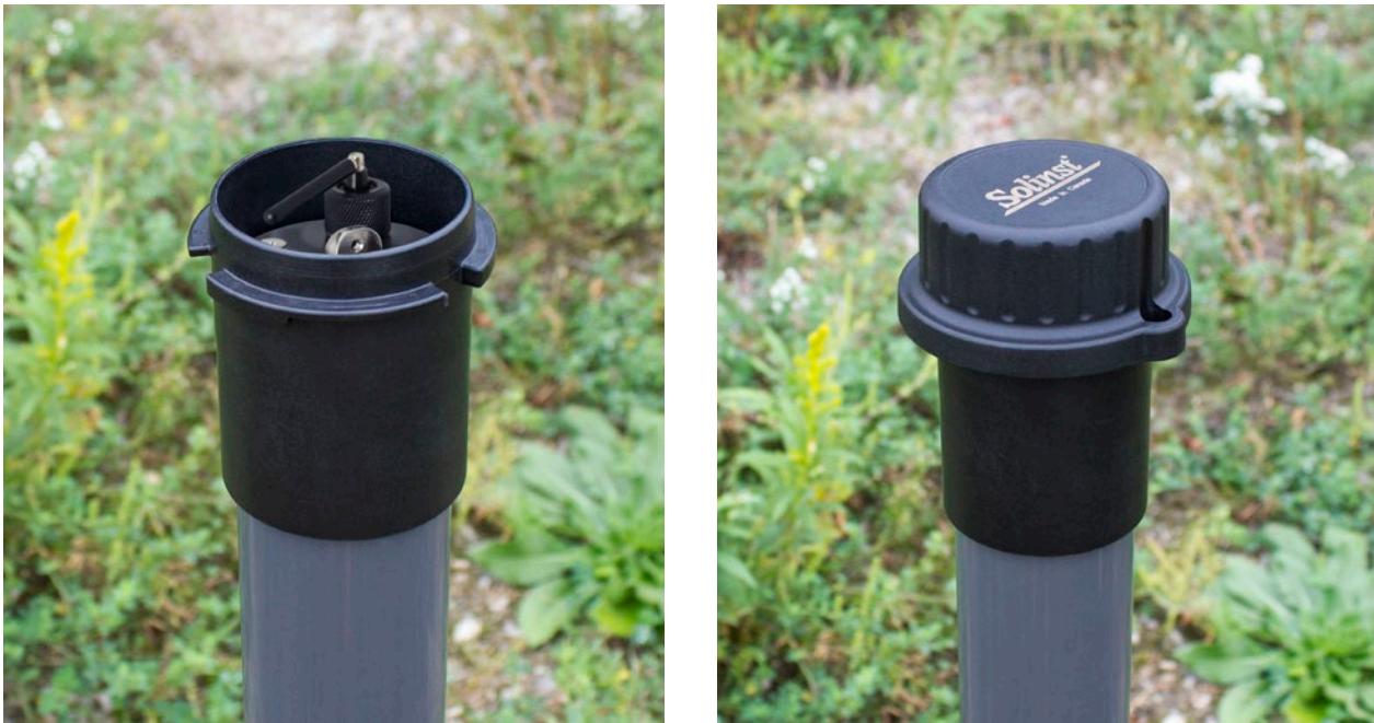
Figure 6-9 Install the Well Cap
