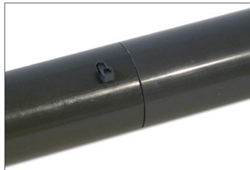
Figure 5-6 Cut Off the Excess Shear Tie
