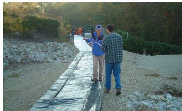
Figure 6-2 Tubing Being Pulled to Reference Mark
