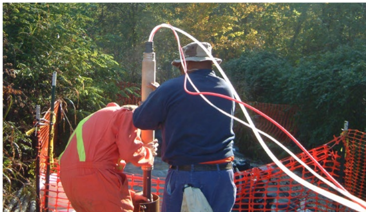
Figure 4-4 Initial Section Being Installed Down-hole
