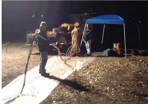
Figure 4-5 Casing Section Being Threaded Over Monitoring Tubing
