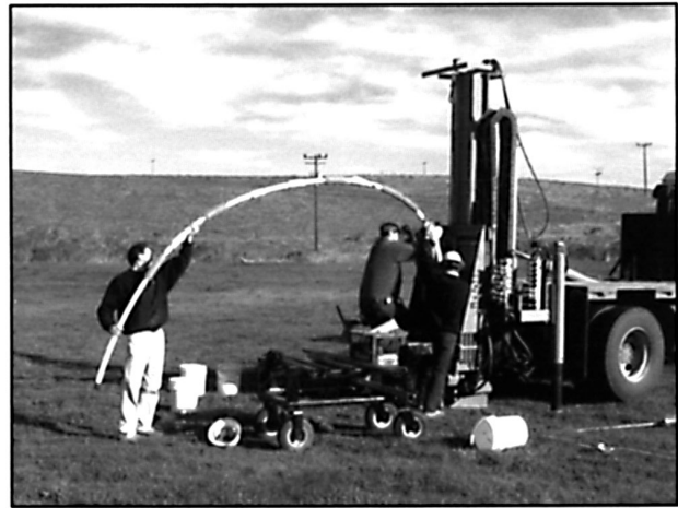
Figure 8. Inserting a CMT multilevel well equipped with bentonite packers and prepacked sand packs.
