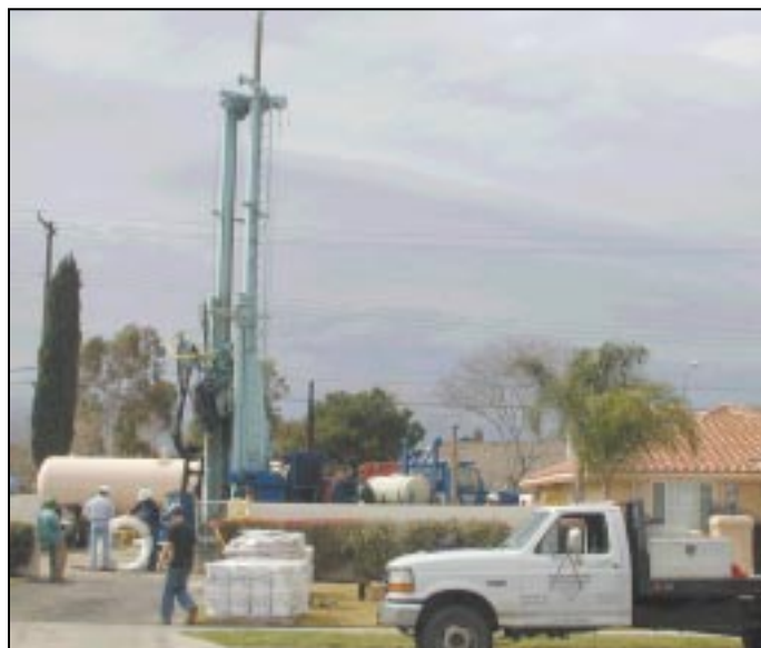
Sonic drilling rig with a bundle of CMT.
