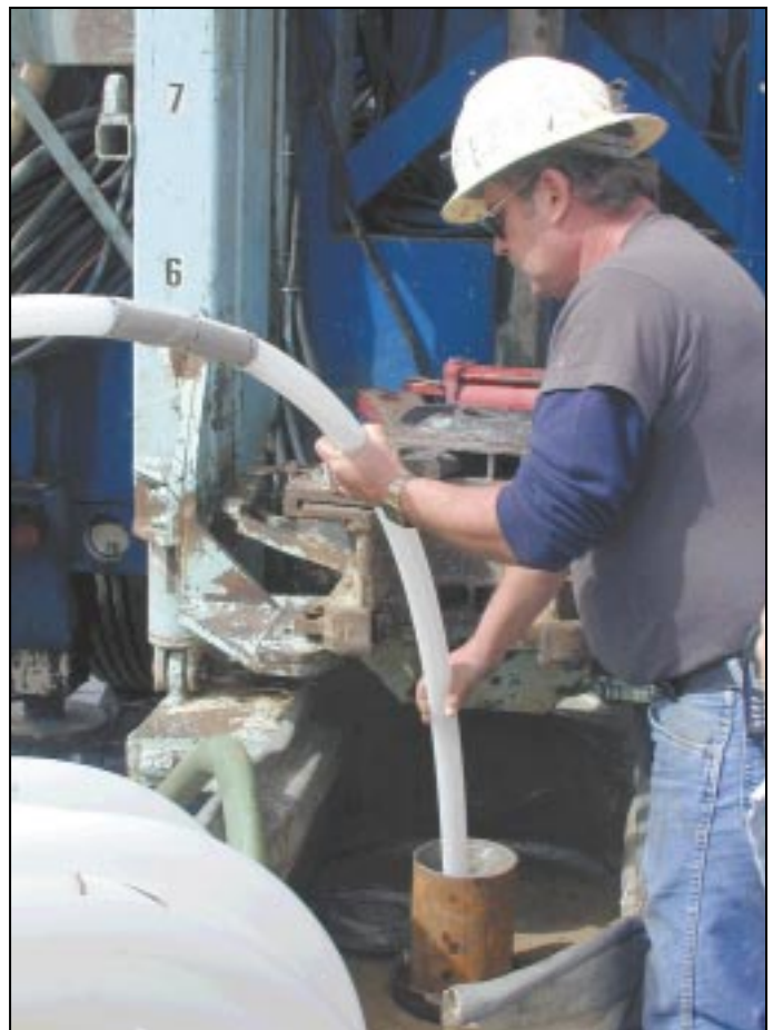
Placing the tubing. Note the screen interval above.
